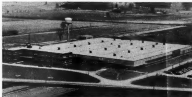
New Lancaster, Ohio, plant of Diamond Power Specialty Corp.
